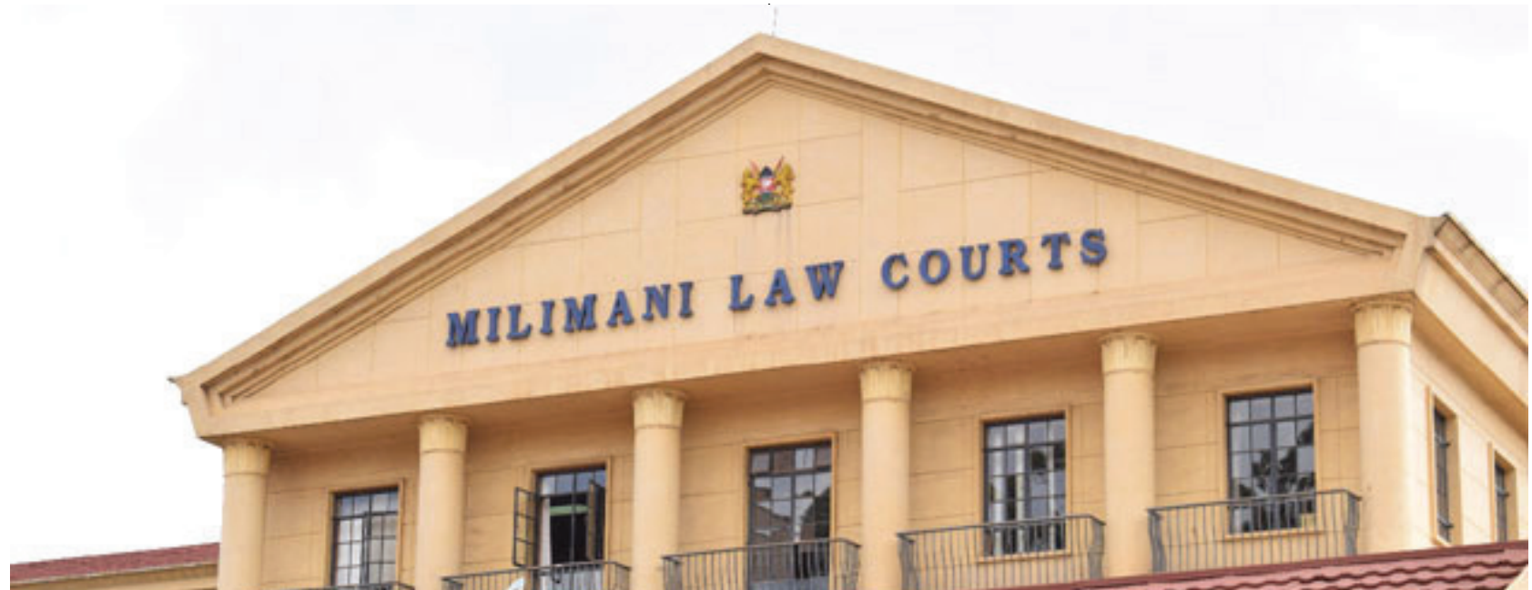
Establishment shot of Milimani Law Courts. Photo Courtesy.
